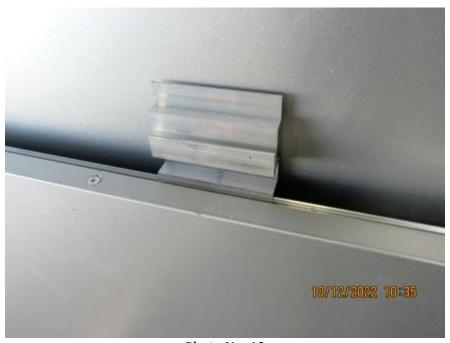
Photo No. 10 Panel clips installed onto panels
