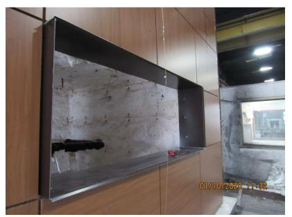
Photo No. 14 Flashing Installed
