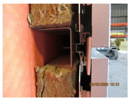
Photo No. 11 Horizontal Joint View
